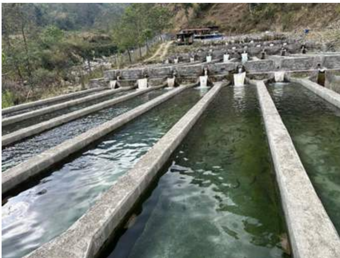
Photo 8: Fish hatchery facility with concrete raceways for aquaculture production.
