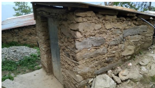
Fig. 7: Toilet constructed with mud mortar in one of the users of Heping W/S Scheme
