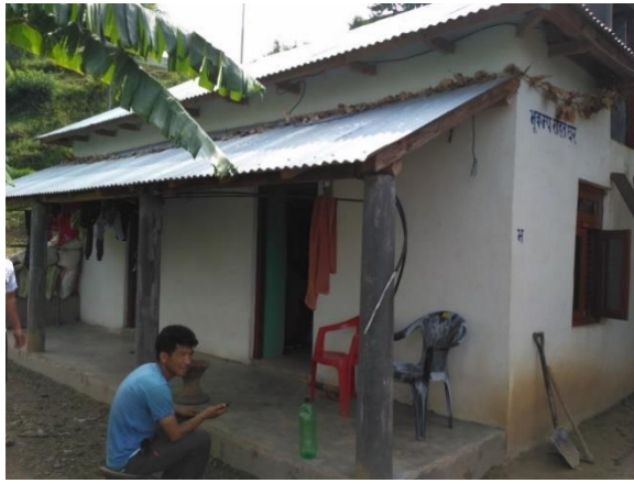
Fig. 5: Proper earthquake-resistant house in rent but house owner is using old house (Makawanpur).
