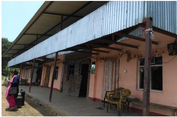
Fig.1: Three Singled room houses of 3 beneficiaries joined by two rooms in between and added hybrid additional floor after receiving all government grant (Makwanpur).
