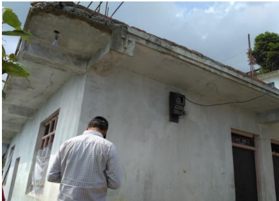
Fig. 6: Some Households are investing in Reinforced Cement Concrete (RCC) structure that is more expensive (Nuwakot).
