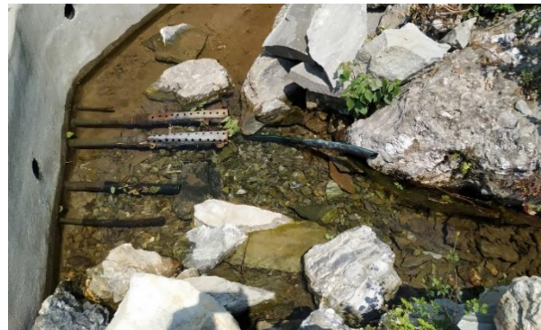
Fig. 6: Water collection pipes at the intake of Heping W/S Scheme (There are 8 different pipes for collection meant for at least 6 schemes, two of them were not fully immersed, the intake design is not up to standard and a source of potential conflict)
