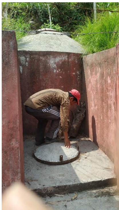
Figure 133 - Reservoir site (Mr. Lama himself removing the manhole cover)
