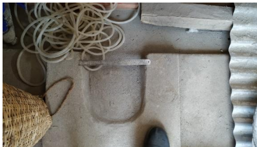
Fig. 5: A Girls urinal (span of squat is 30 cm) in Nuchet Primary School, Nuchet, Bhalche. The toilet was constructed under American Red Cross and Spanish Red Cross
