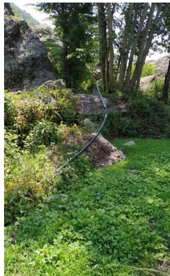
Fig. 10: Transmission line of Heping W/S Scheme (HDPE pipes should be avoided in exposed or rocky area)
