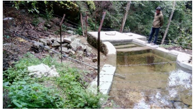
Fig. 20: Intake of Jantare Khola W/S scheme, Thaha -5, Makawanpur (A GI pipe on the left seems unusual and the fencing without cross line
