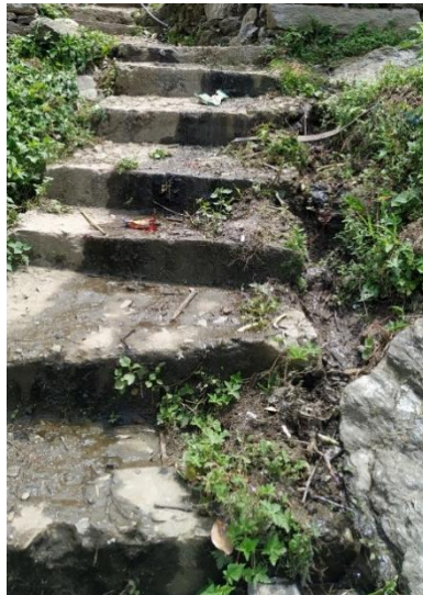
Fig. 11: Poor drainage of the wastewater from the tap leading to the flooding of walkway and pollution at the project area of Heping W/S Scheme
