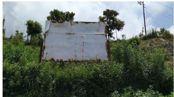
Fig. 12: Poorly maintained Hoarding Board of Heping W/S Scheme
