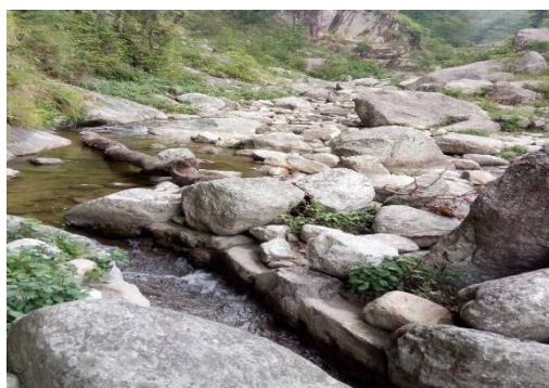
Fig. 1: Intake site of the Duwa Khola Irrigation Project, Gogane-8, Makawanpur
