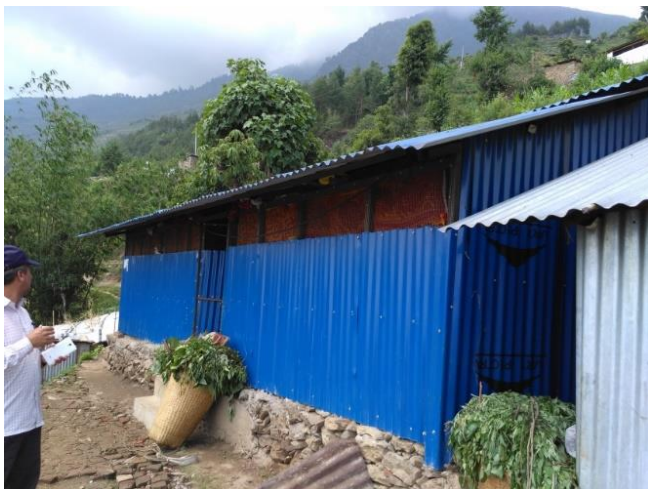
Fig. 7: The reconstructed house cannot be seen due to temporary construction around the house in Rasuwa.
