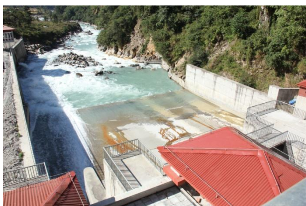
Downstream of weir structure of Upper Marsyangdi A
