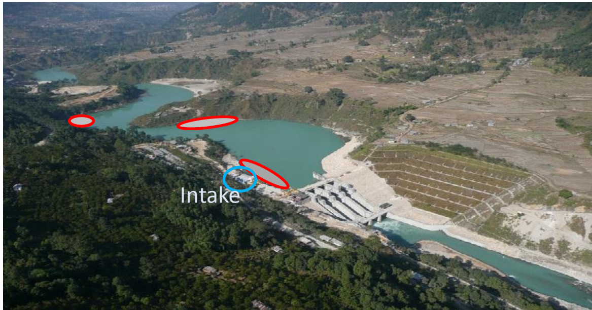
Figure 2-7: Areas of high sediment deposit upstream of the reservoir (red marked areas) and location of intake (blue marked area), (Source: NEA , 2016 b)
