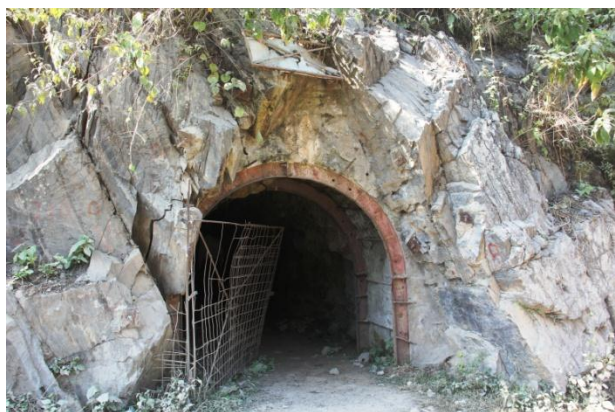
Test Tunnel at Budhi Gandaki HEP Dam Axis
