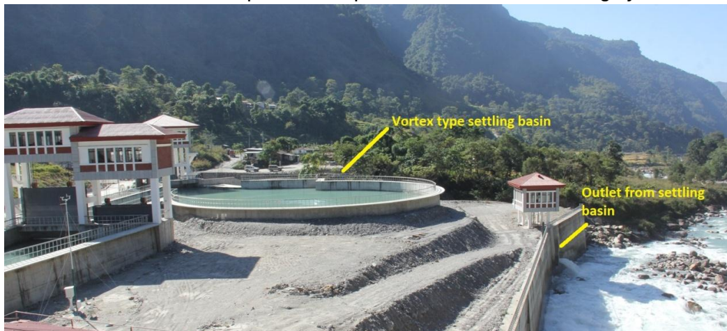
Figure 2-3: Vortex settling basin and its outlet in Upper Marsyangdi A Hydropower project
