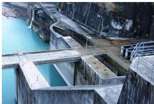
Weir Structure of Middle Masrsyangdi HEP
