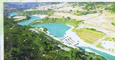
MMHPS Dam and Reservoir
